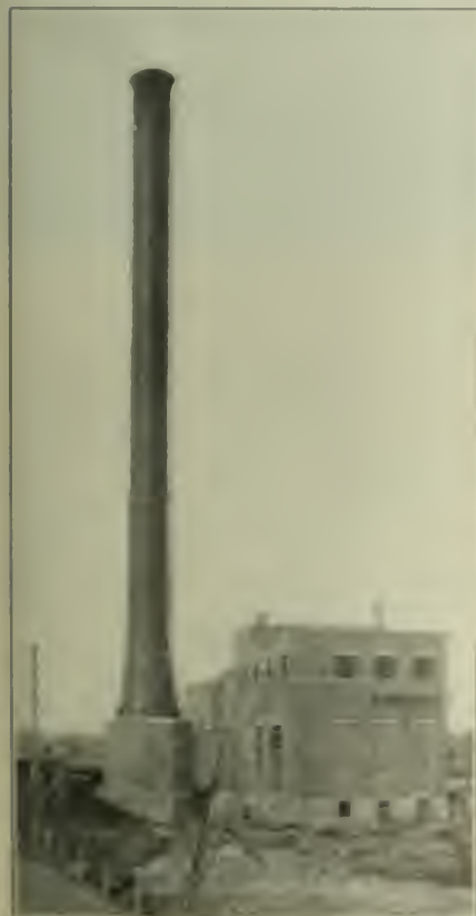
FIG. 1. TURBINE STATION AT EAST BRIDGEWATER.
